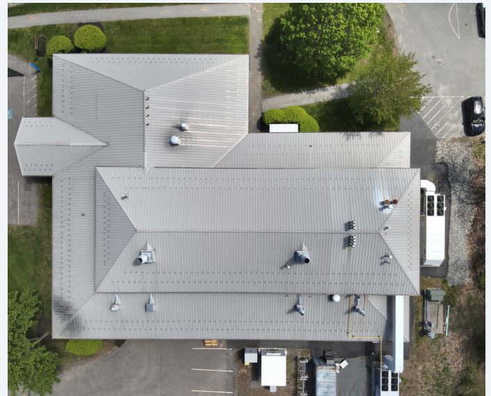
Aerial Drone Imagery of the Teaching Laboratory
