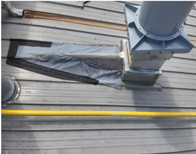
Split Base Flashing on the Teaching Laboratory
