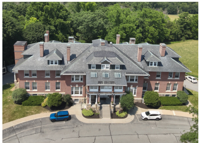
Aerial Drone Imagery of the Administration Building
