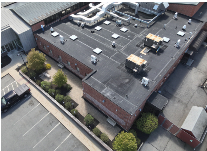
Aerial Drone Imagery of the Small Building
